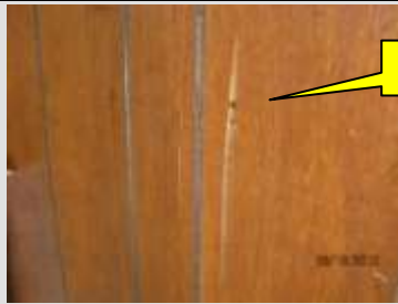
Delaminated siding
